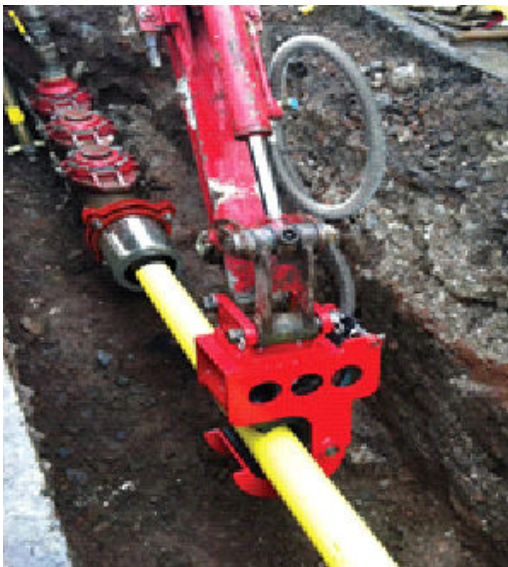
Entry pit pushing 4" PE into 6" cast iron
