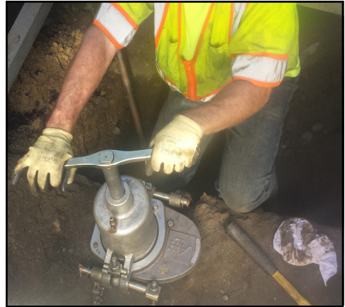
Plug removed. A special rubber stopper inserts into the tee stopping the flow of gas.
