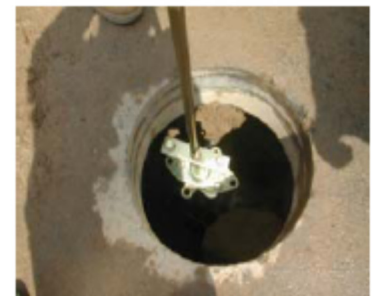
Installing a 1 1/2" Low-Profile Plug
