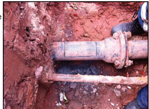
Circumferential and Longitudinal Cuts
