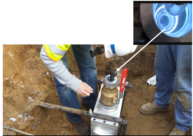
Viewing the main hole with the Safe T Stopper prior to inserting the correct size Self Tapping Plug.
