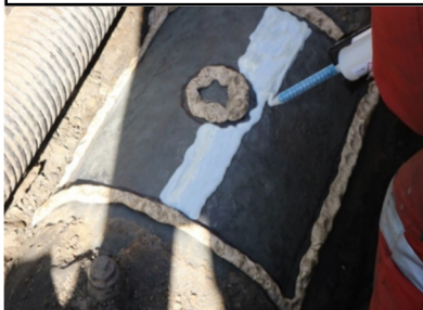
1. Clean work area and apply adhesive.
