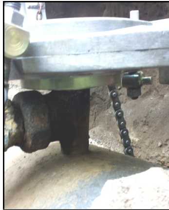
Equipment creates a seal on top of the tee.
