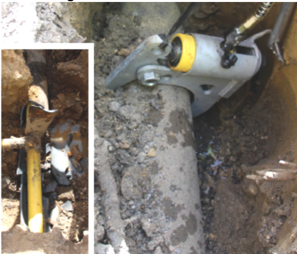
Cracking a section of 4" cast iron main.
