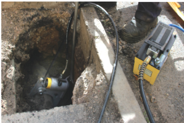
Cracking a section of 4" cast iron main.
