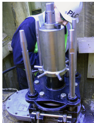
Drill Head Attached to Valve (Air Motor slides down the guide bars)
