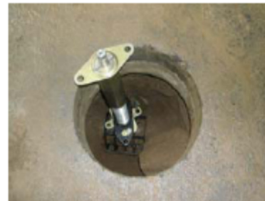
Cut and Tap an 1 1/2" Hole (Note large obstruction)
