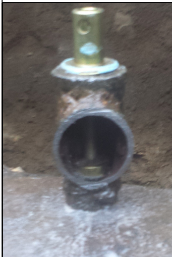
Seal is locked into place. Branch is cut.
