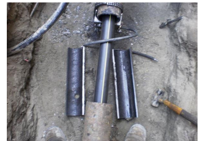
Circumferential Cutter Module
