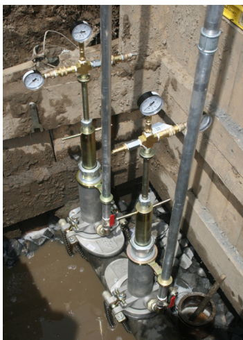
Simple Double Block and Bleed Operation
